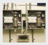
Two Excel 10<sup>™</sup> Constant Volume Air Handling Unit Controllers (W7750C2001) provide cost-effective control of constant volume single-zone air handling units and heat pumps. Part of the Honeywell Light Commercial Building Solution<sup>™</sup>, CVAHU Controllers work with a LonWorks<sup>®</sup> communications bus or in standalone applications, providing reliable and affordable control.
