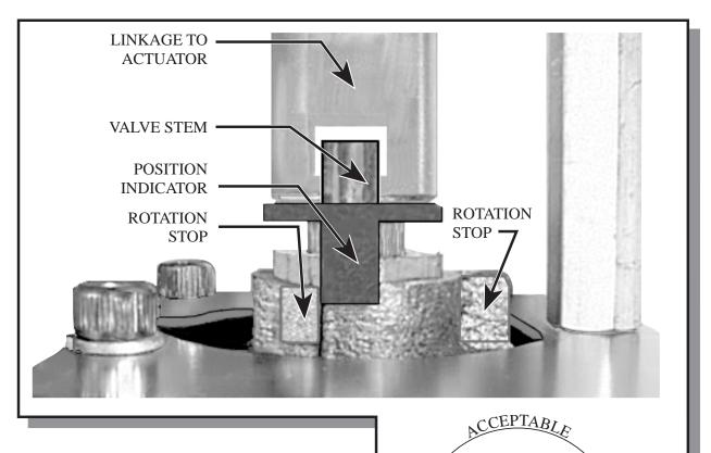
Most ball valve stems are either 1/2 (13 mm) or 1 inch (25 mm). The hub size of the actuator should match the diameter of the stem. This is important since most of the direct coupled actuators are available with various hub sizes. Similar to most globe valves the stem should always be one degree or more above horizontal. Direct contact of moisture or condensation can cause damage to most direct coupled actuators.
