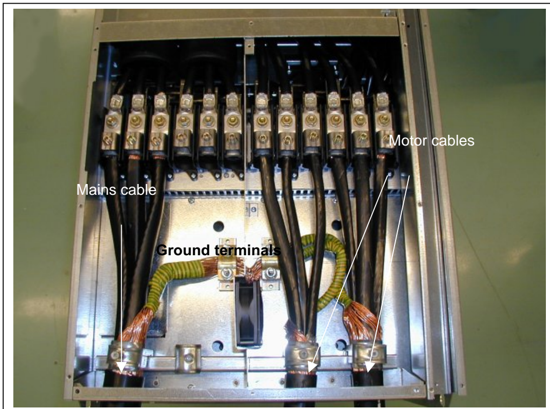
Figure 6-19. Cable installation in NX, FR9
