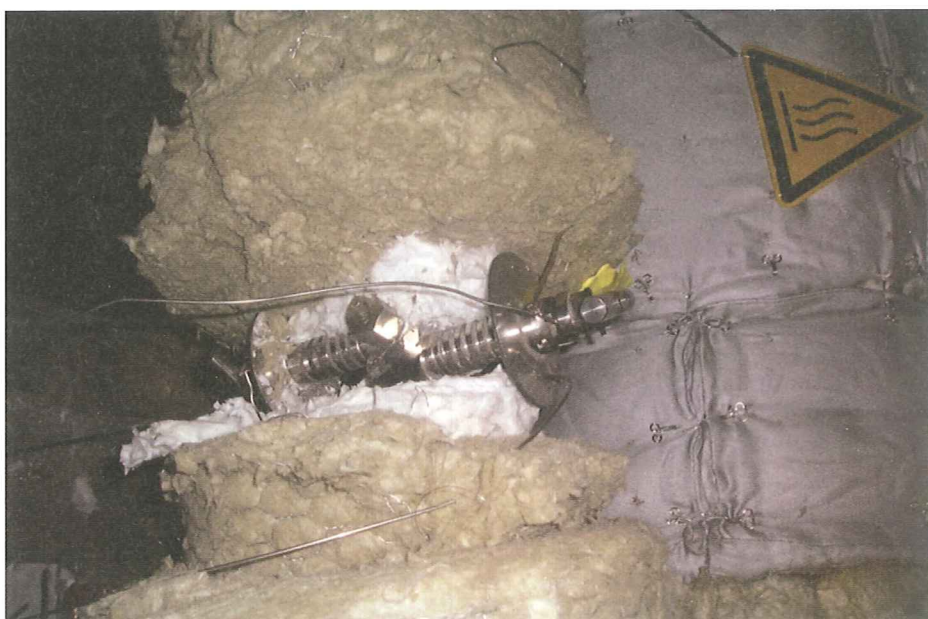
AS-Schneider dual shut-off valve installed in a test plant COMTES700 for a long-term design test.
